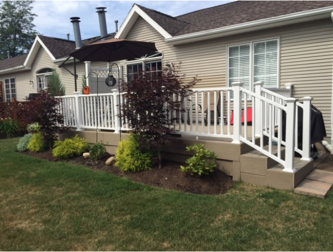
This is an example of a deck that has been replaced with composite decking and vinyl railings
