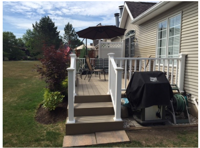
This is an example of a deck that has been replaced with composite decking and vinyl railings
